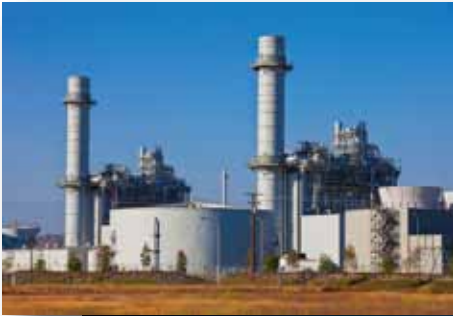
● Nature Gas Fired Power Station
