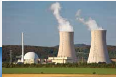
● Nuclear Power Station
